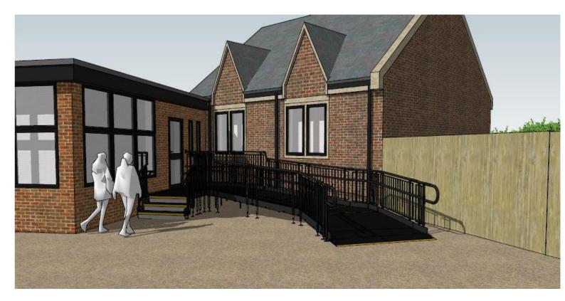
**END RESULT:** The Rapid Ramp included a 1:15 gradient and fully complies with <u>documents M & K of the</u> <u>building regulations.</u>
