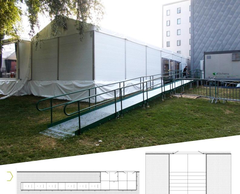
**END RESULT:** A Rapid Ramp and step unit were manufactured, designed, and delivered to site, ready to be assembled.
