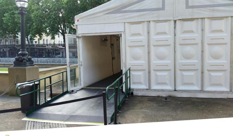
END RESULT: Our installation team installed two heavy-duty framed Rapid Ramps from the entrance and exit with slip-resistant GRP platform.
