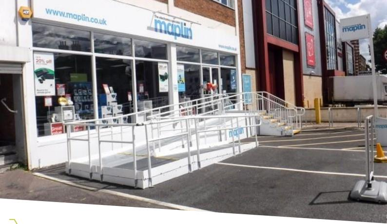
**END RESULT:** A modular Rapid Ramp and step unit replaced the existing steps. The systems were powder-coated white to colour match the building.
