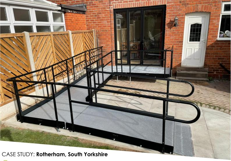
REQUIREMENT: A modular ramp design that could easily accommodate the width of the bi-folding door and provide enough room for a wheelchair to turn.
