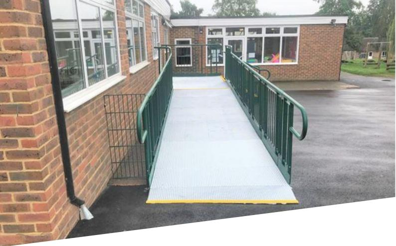
**END RESULT:** Once the new door was fitted, we installed a fully compliant Rapid Ramp with step unit. We were able to achieve the necessary finished floor height with adjustable telescopic legs.
