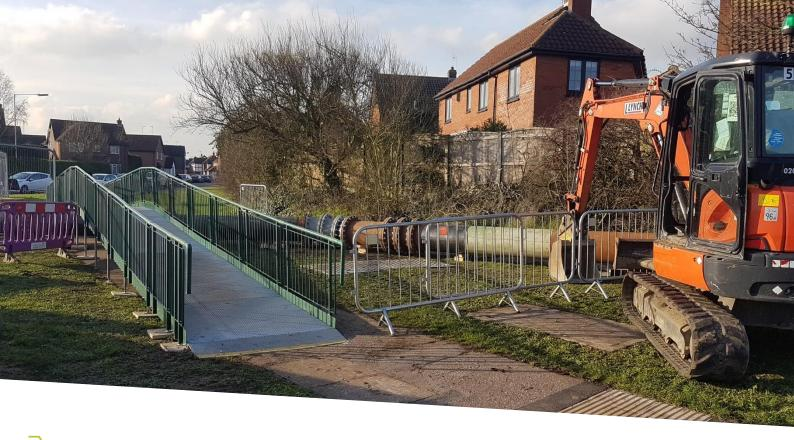
END RESULT: Three Rental Ramps were installed prior to the repairs, and the pipes were moved into place underneath.
