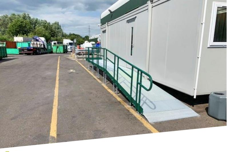
**END RESULT:** We designed and installed the ramp by the deadline. Only a single handrail along one side was necessary, to prevent encroaching on the walkway.
