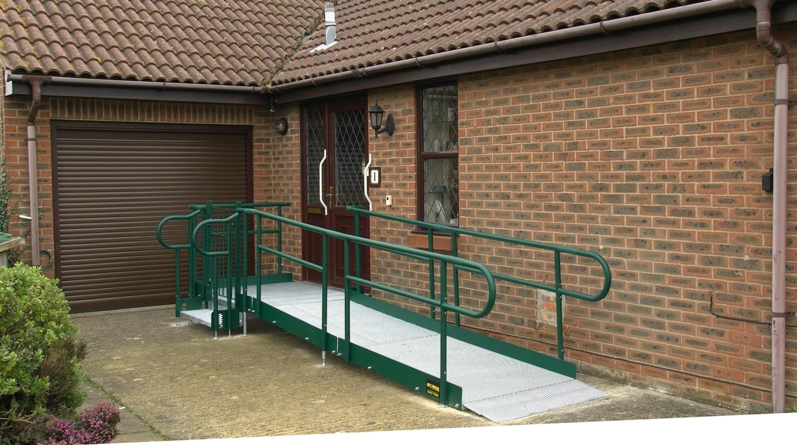
**END RESULT:** Our team installed the Rapid Ramp with a step and gate unit within a few hours.
