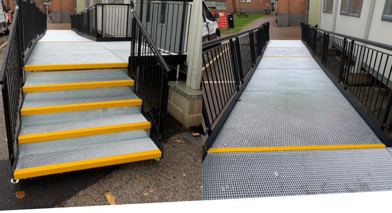
**END RESULT:** Once the building had been assembled, we installed a fully compliant Rapid Ramp with step unit from the front entrance.
